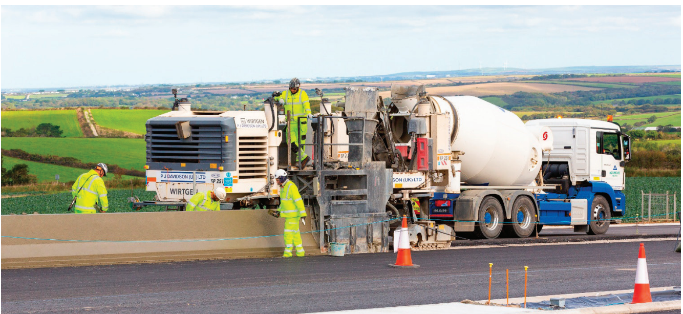
Fast installation of RCB barrier. Photo credit PJ Davidson
